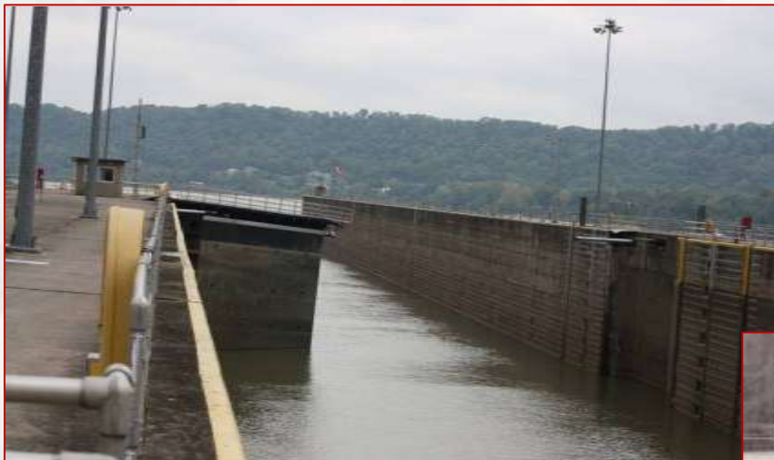
Greenup main chamber gate dropped when anchor point failed >
