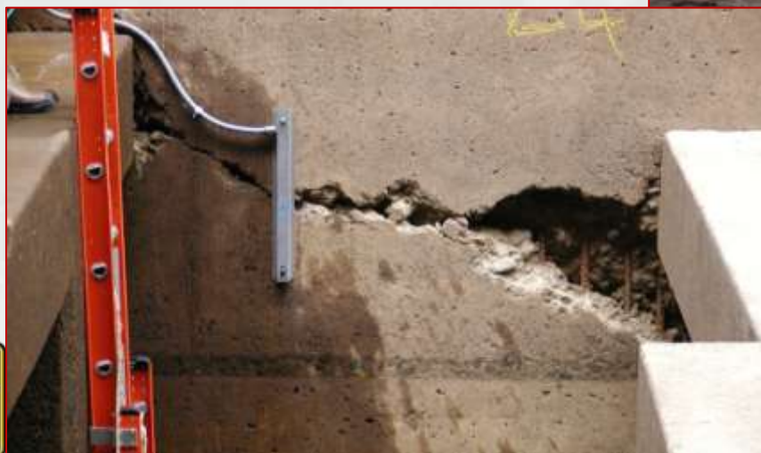
< Monitoring of decaying sidewalls of John Day lock
